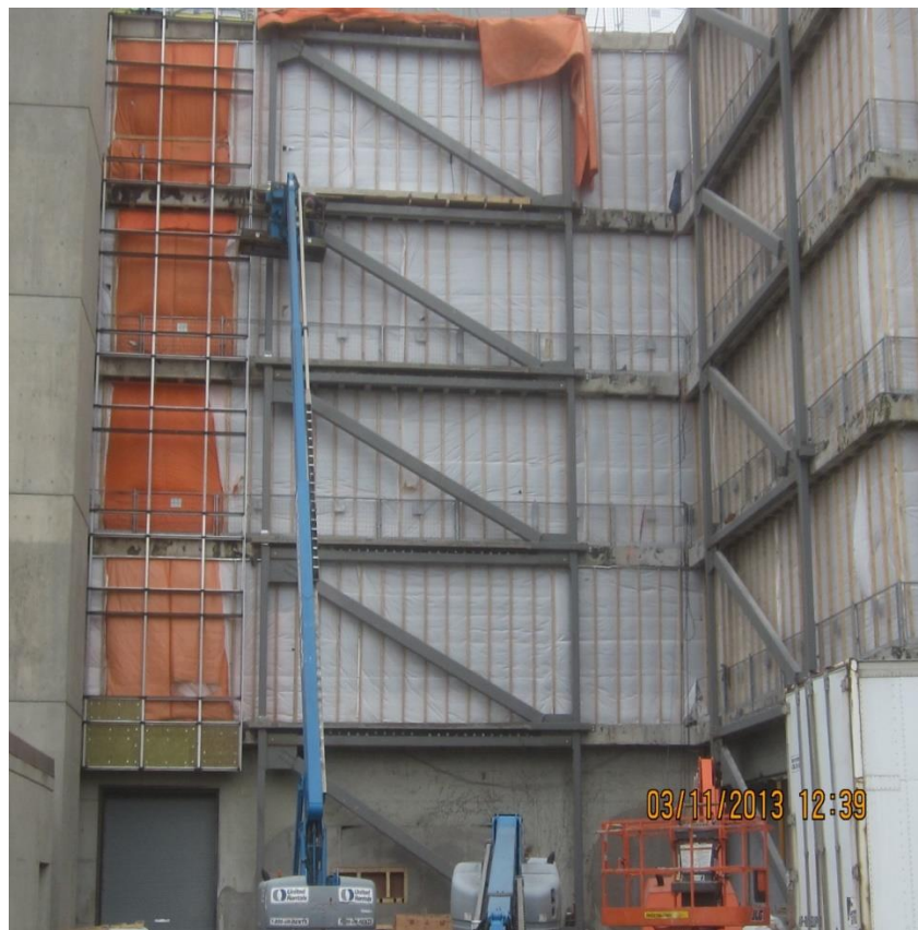
Figure 5. Seismic bracing added to the exterior walls of Sawyer Mod 5 during 2012-2013 renovation.
